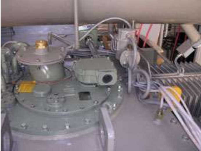
16 MVA kV 33 ± 9X1,25% COPERCHIO - COVER
